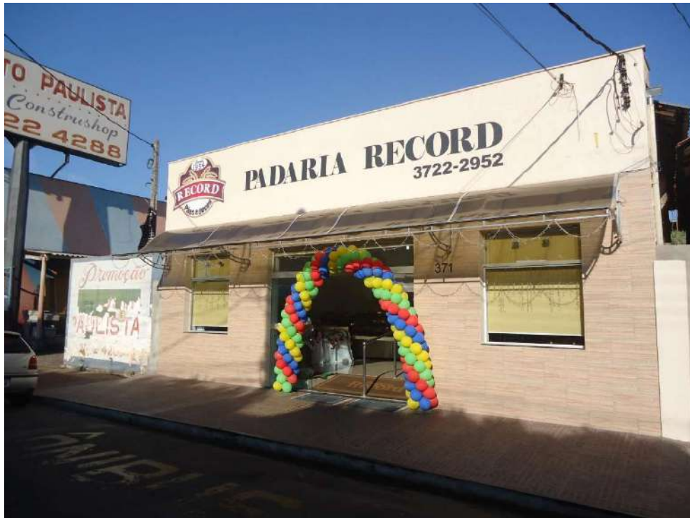
Figura 117 – Padaria Record - Fachada
